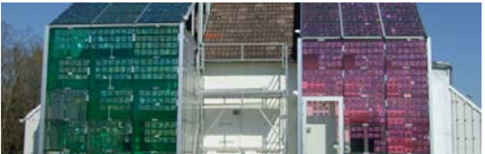
Prototype double peau photovoltaïque, ETI Construction, 2015
